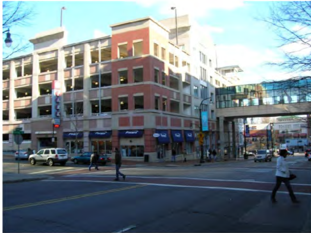
Figure 1: Example of parking structure with integrated architectural treatments and with ground-level retail space.
